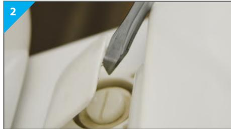
2 Next, place a screwdriver on one of the mounting bolt heads. Firmly holding the corresponding nut (underneath the toilet base), turn the screwdriver anti-clockwise to loosen.
