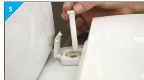
5 Align the holes of the new seat with those of the toilet's base. Push the mounting bolts through the holes. Screw on the nuts from underneath until hand-tight.
