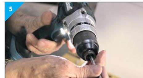
5 Replace your diamond core drill bit with a masonry one. Be sure to turn off the hammer action. Start drilling slowly.
