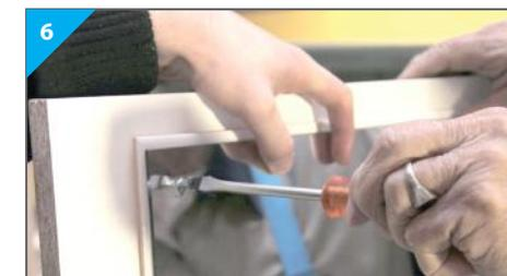
6 Insert all four wall plugs into the holes in the wall. Make sure they fit. Insert the nylon plugs into the mirror. These will fasten to your wall plugs. Using all the wall screws, secure your mirror to the wall. To finish the job, attach chrome caps to the end of each screw. That's it!
