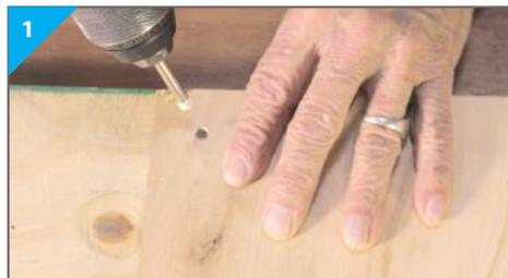
1 Cut a plywood board to match the measurements of your mirror. Drill a hole through a corner of the board using the same size drill bit for the wall. This hole will act as a guide.
