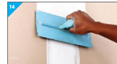
14 Apply a second coat off Rhinoglide using a 300mm steel trowel.
