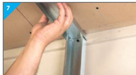
7 Insert top UltraSTEEL® Track into position.
