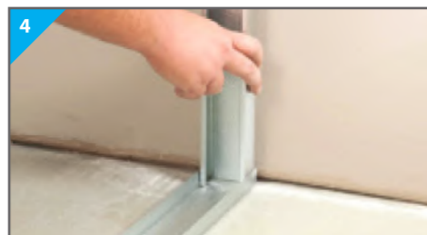
4 Twist Donn UltraSTEEL® Stud into place.
