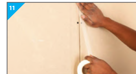
11 After the boarding is complete, apply Gyproc RhinoTape to all joints.
