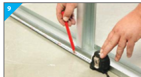
9 Insert UltraSTEEL® Studs at 600mm centres to a friction fit within the channel sections – this allows for adjustment during boarding. Position the UltraSTEEL® Studs so all face the same way.
