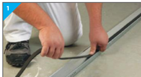
1 Apply SoundSeal as a continuous application to the perimeter of the framework.
