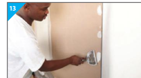
13 Fill all screw heads using Rhinoglide.
