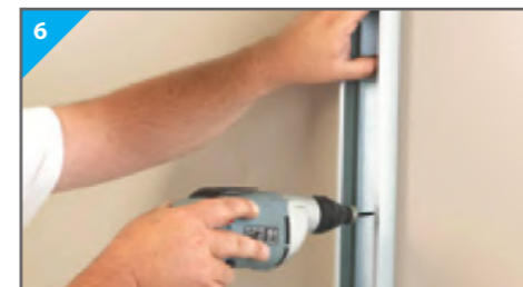
6 Fix the UltraSTEEL® Stud to the abutting wall at 600mm centres using suitable fixings.
