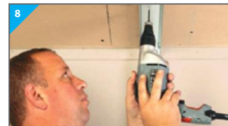
8 Insert top UltraSTEEL® Track into position.
