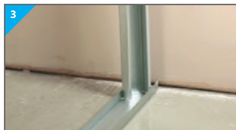
3 Measure the wall height and cut stud to size. Install the stud into Donn UltraSTEEL® Floor Track.
