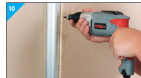
10 Fasten Gyproc RhinoBoard 12.5mm to the framework using Gyproc RhinoBoard Sharp Point Screws 25mm spaced at 220mm centres.
